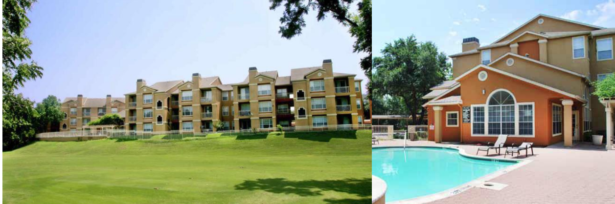
Laguna Luxury Apartments view overlooking golf course (left) and poolside (right)
